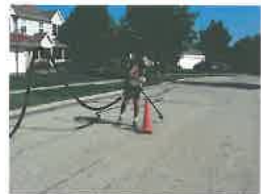
The crack is sealed using a hot applied rubberized sealant.
