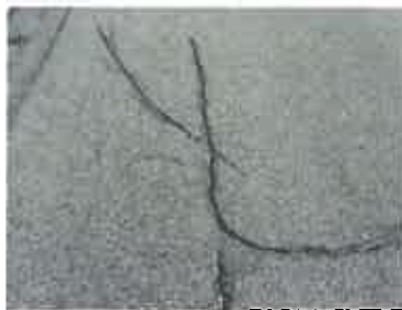
The crack is sealed using a hot applied rubberized sealant.
