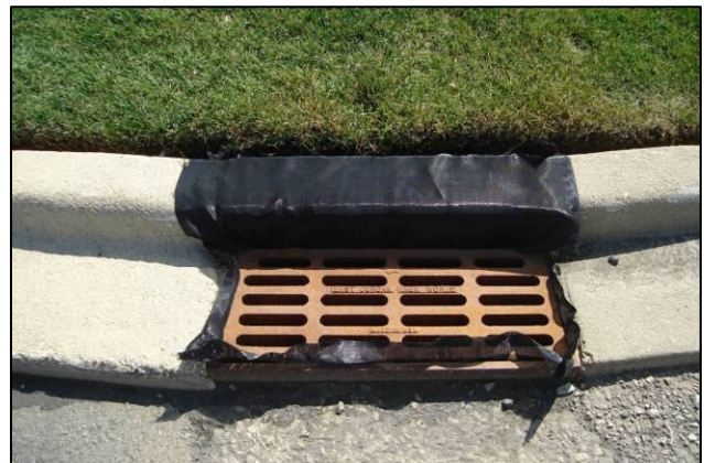
Example: Sedimentation control installation
