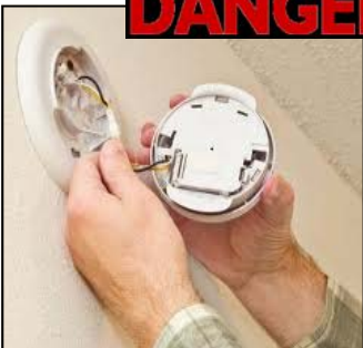
Hard-wired Smoke Detector
