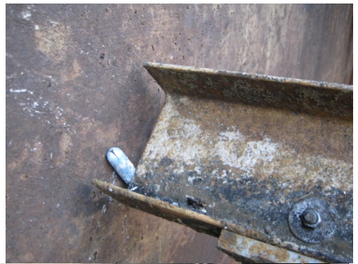
Work on flight repairs
