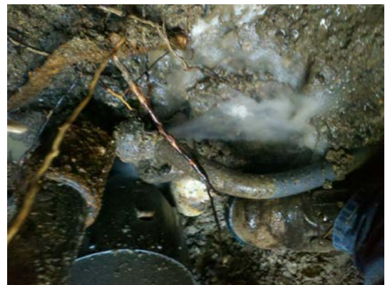
Leaking b-box
