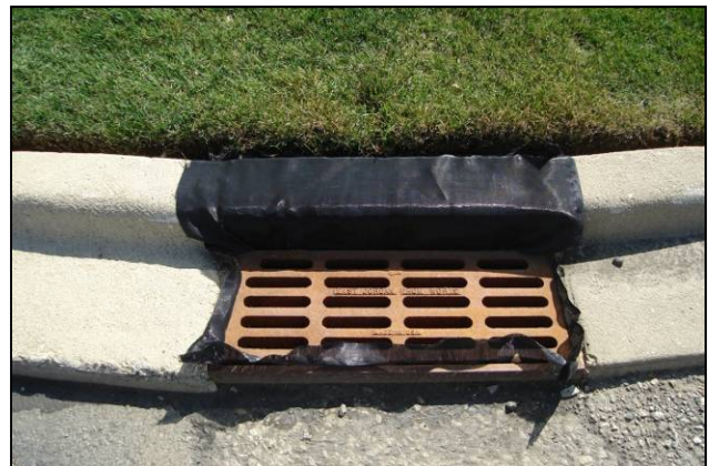
Example: Sedimentation control installation
