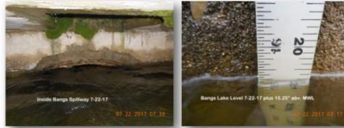
Spillway Drain Pipe maxed out when the lake level reached plus 15.75" on July 22, 2017
